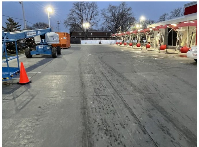
Tommy's Car Wash — Completed
