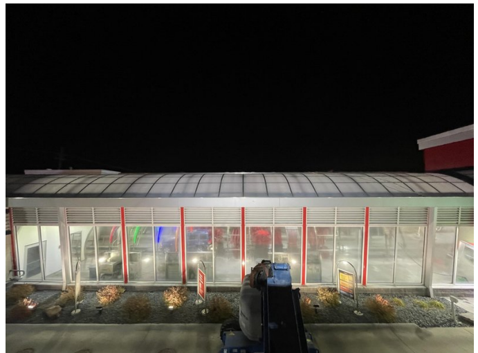
Tommy's Car Wash — Exterior Completed
