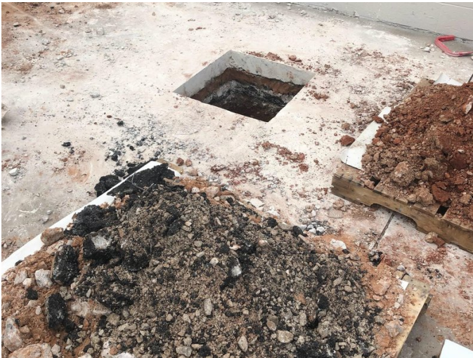
Concrete Core Demolition
