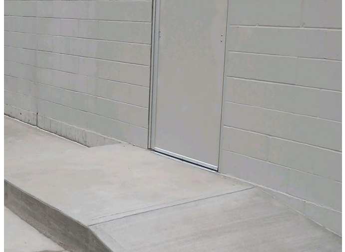
Door Frame — Completed
