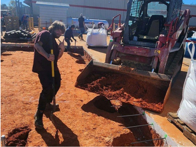
Foundation Excavation & Prep
