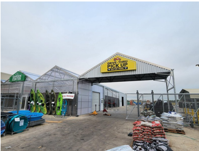
Tractor Supply — Drive-Thru Pickup Construction
