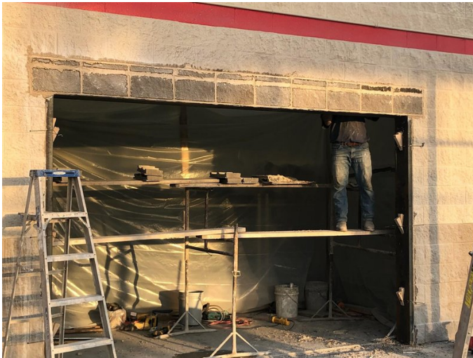
Exterior Wall Opening — In Progress
