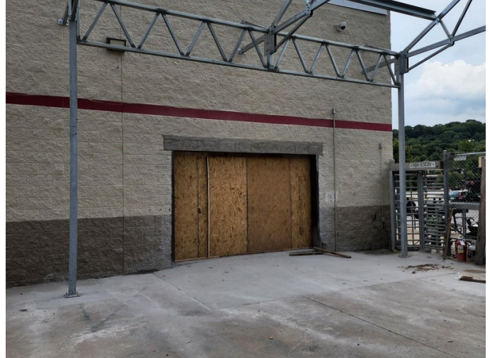
Tractor Supply — Canopy Construction
