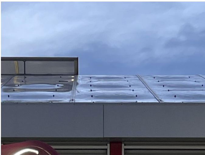
Tommy's Car Wash — Exterior Construction
