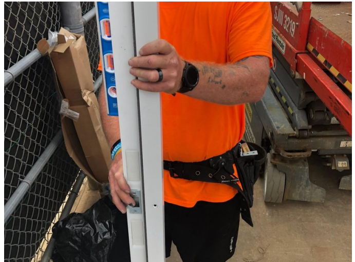
Security Fence / Gate Install
