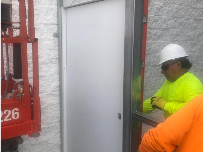
Fixture & Door Installation — Rollout Program
