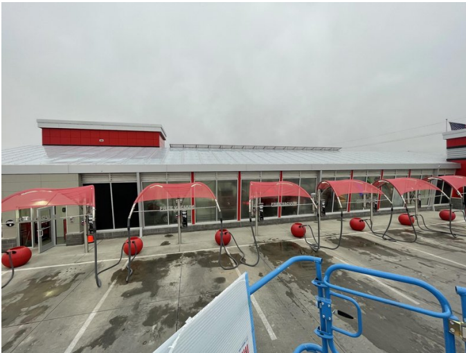
Tommy's Car Wash — Site Work
