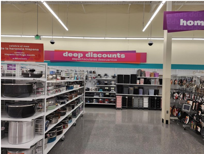
High-End Retail Interior — Fixture & Shelving Install
